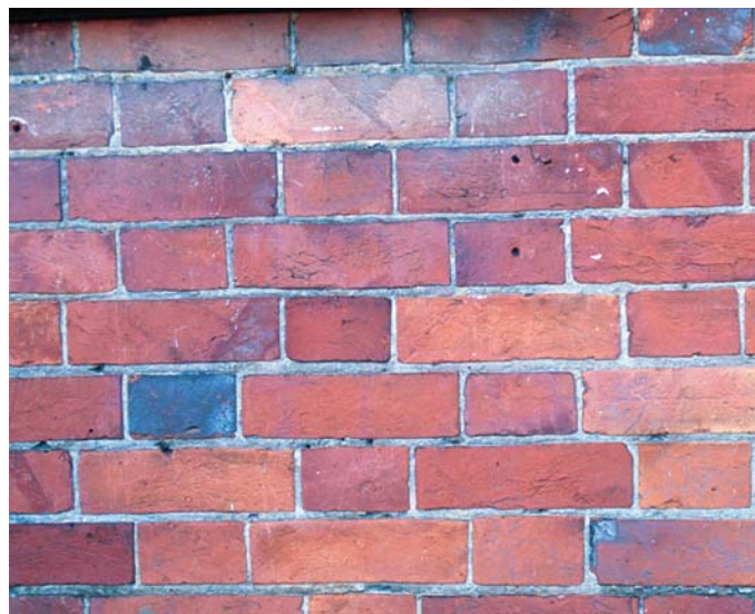
Flemish-bond brick work
