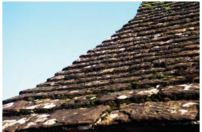
Horsham stone slab roof
