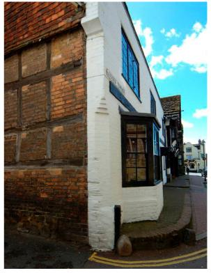
Fig. 15. 1-2 Judges Terrace, High Street: 18<sup>th</sup>-century façade applied to mid-15<sup>th</sup>-century timber framing.
