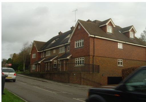
Discreet underground parking at Springfield Shaw
