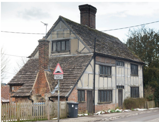
Casteye Barn - one of the earliest houses in the village with stone roofing and timber cladding. Brick and stone is used only for chimneys and at foundation level.
