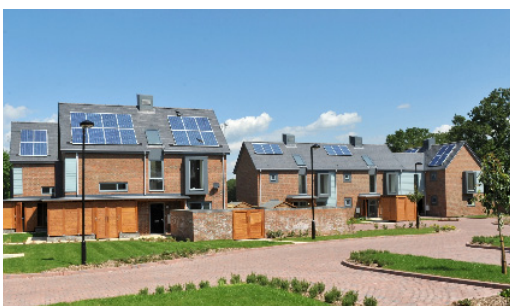
Crawley Down affordable housing - a development by Hastoe which featured in Inside Housing Top 50
