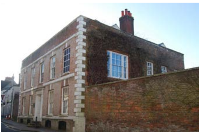
Photo 9: Mansion House, the High Street. This 17th century or earlier timber framed building was refronted in the early 18th century.
