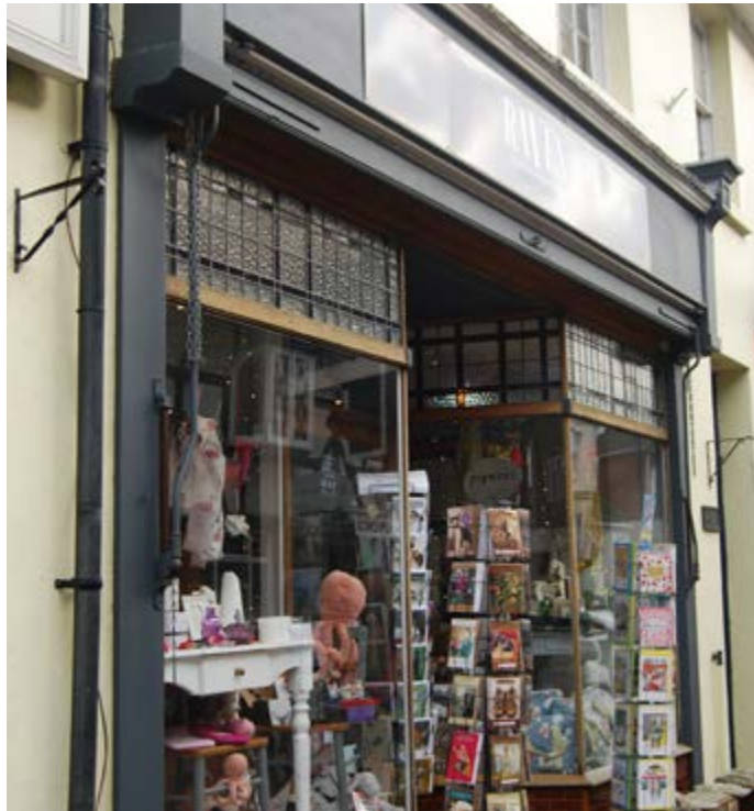
Photos 60, 61 and 62: Architectural features of shop terraces on the High Street
