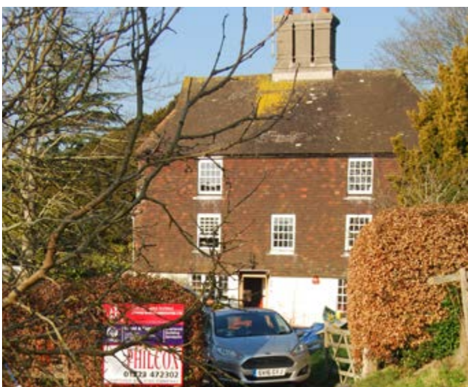
Photo 7: Tott Farmhouse, Tott Lane- a 16th century three storey timber framed house, refronted with stucco and tile hung.
