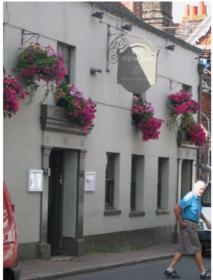
Photo 59: The New Inn
