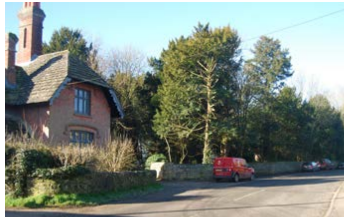
Photo 126: The stone and flint wall with overhanging trees along the frontage to Pakyns Manor
