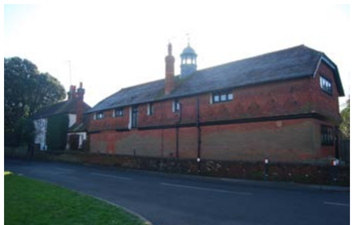
Photo 121: Littlemead and Paddock Cottage, formerly part of Grange Farm, turn their backs on the road.
