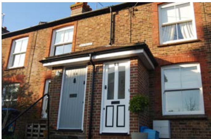
Photo 112: Porch additions detract from the appearance of the terraced cottages
