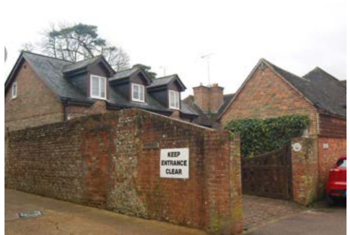
Photo 95: The former printworks at the western end of West Furlong Lane.
