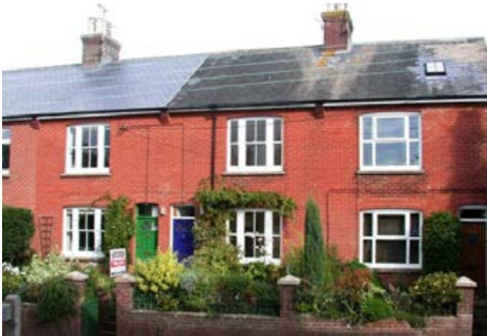
Photo 111: Tripartite sash windows to houses on College Lane
