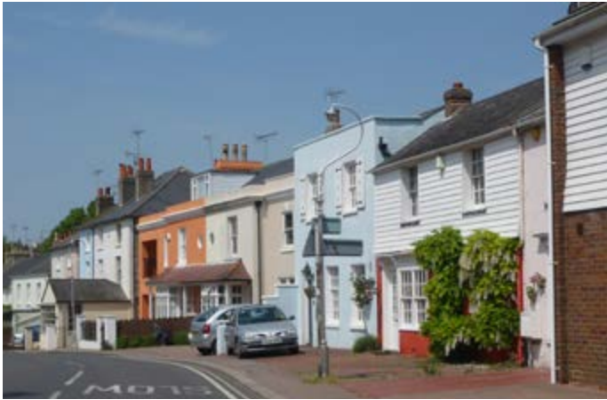
Photo 24: Tightly packed cottages line this part of the High Street
