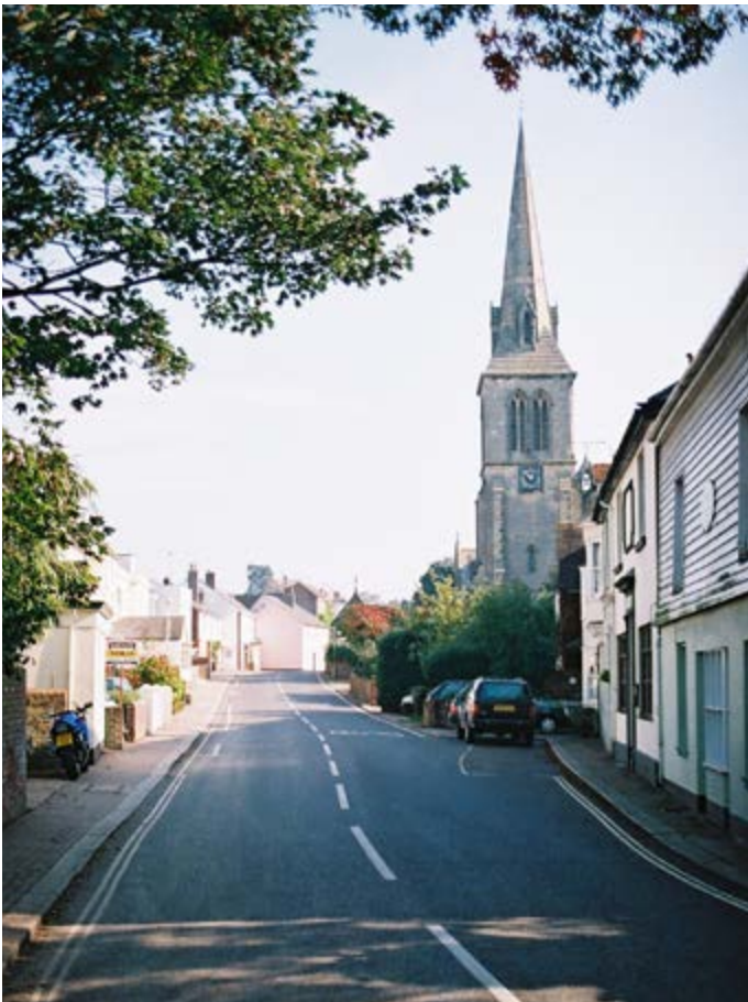
Photo 22: Holy Trinity Church is prominent in views looking east along the High Street
