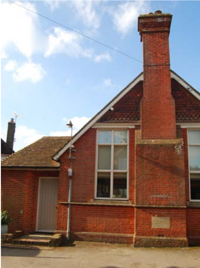
Photo 96: The former Parish Rooms, built in 1890
