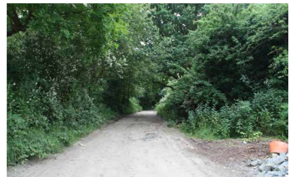
Site visit photos from Freeks Lane
