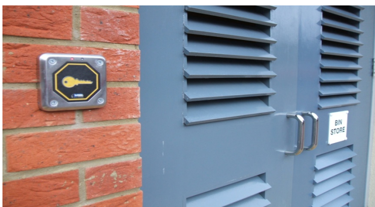
Photo 3. Example of good practice - bin store lock.
