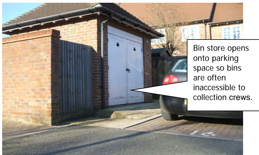
Photo 4. Example of bad practice - inaccessible bin store.
