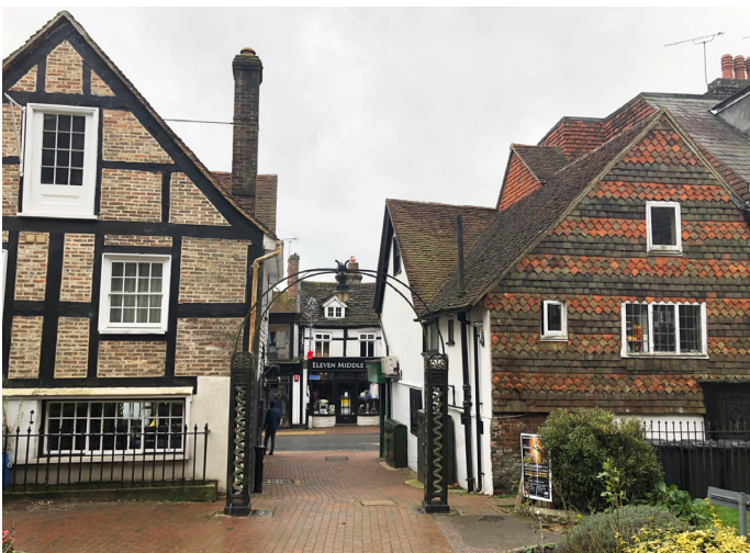
View South from Church of St Swithun
