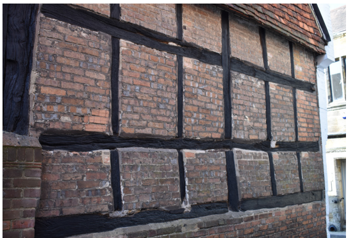
Brick infill panels to side of 1-2 Judges Terrace
