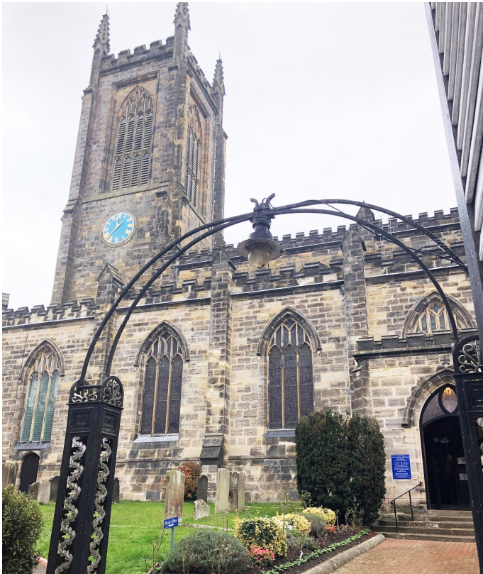
Wrought iron gate piers and archway to Church of St Swithun
