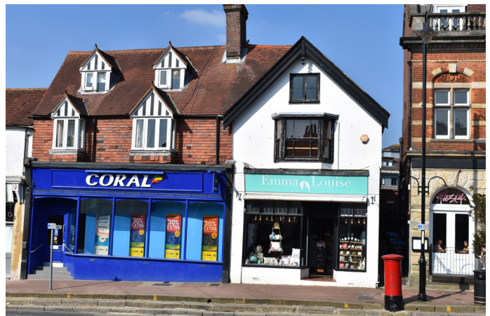
7 - 9 High Street: Negative shopfront - oversized fascia and garish paint colour
