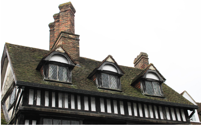
Dormers on Cromwell House, 80 High Street
