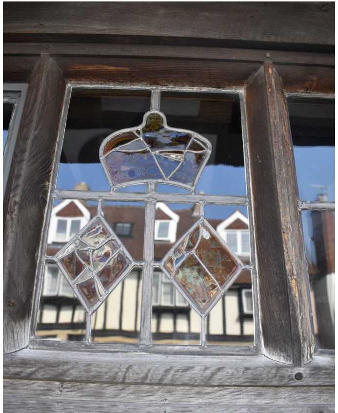
Leaded-light timber window - Cromwell House, 80 High Street
