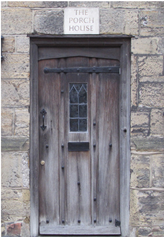
Oak door with iron detail of The Porch House, 82 and 84 High Street
