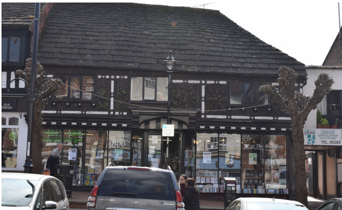
Tudor House, 22 and 24 High Street
