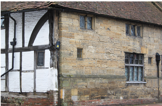
Timber framing and sandstone wall of 84 High Street
