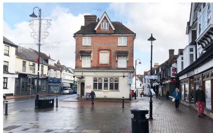
View of the Former Midland Bank, from West of High Street
