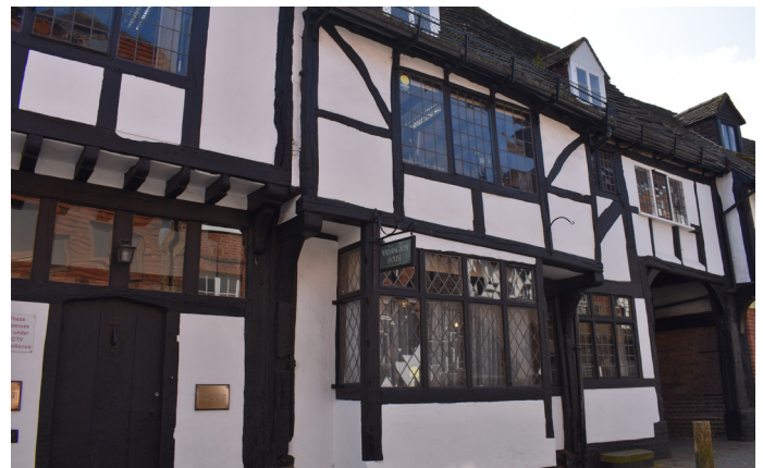
Wilmington House, 48 and 50 High Street
