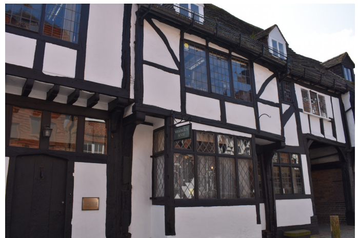
Wilmington House, 48 High Street
