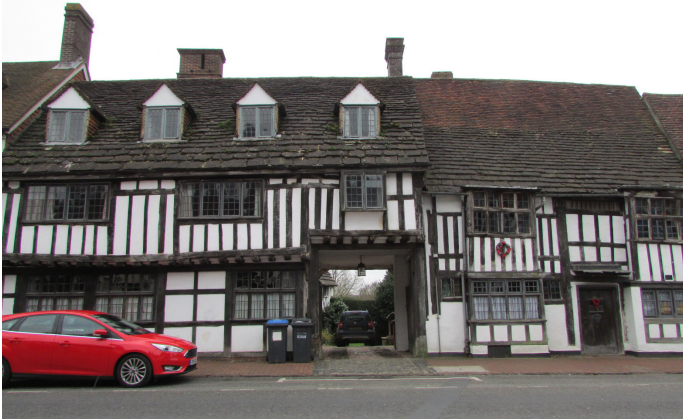
Sackville House and Amherst House, 66-72 High Street
