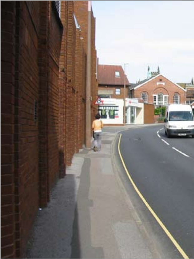
West Street presents blank walls.
