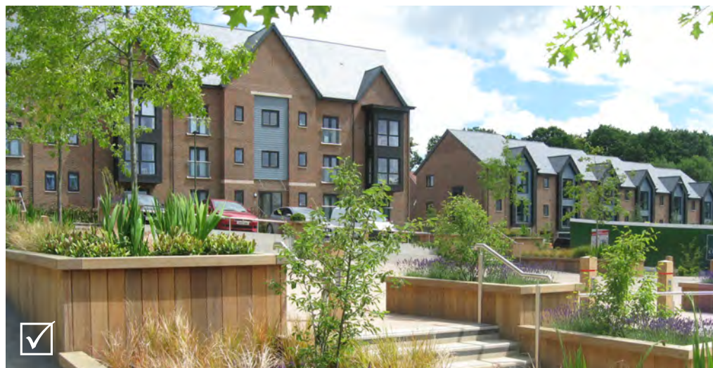
The central square in Kings Weald, Burgess Hill to be defined on all sides by public facilities including a shop, community centre and health centre
