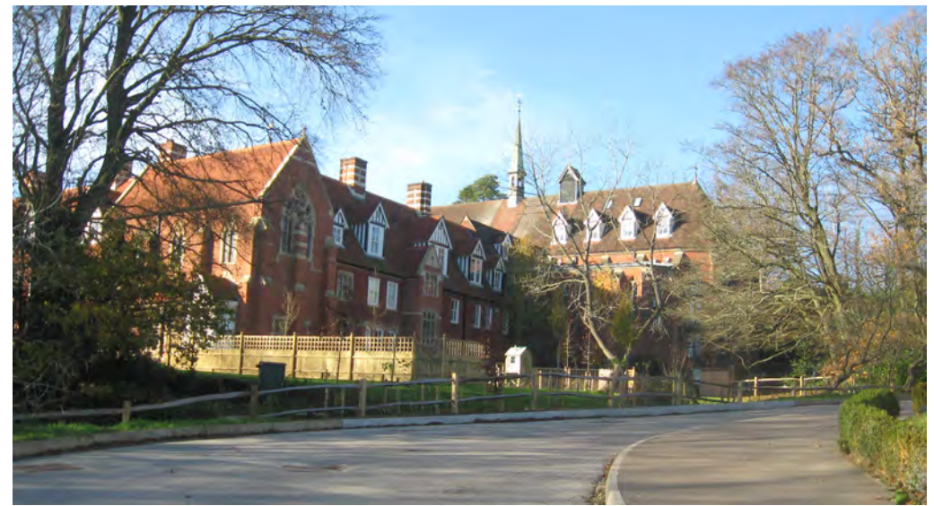
The former convent at Grosvenor Hall in Haywards Heath has been sensitively converted to residential use
