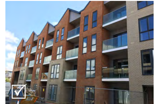
A recent higher density scheme in East Grinstead town centre which has reduced its apparent scale by employing consistent vertical articulation
