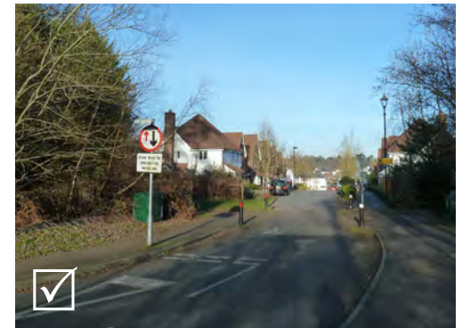
Controlling traffic speeds through road narrowing at Bolnore, Haywards Heath
