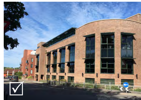
The curved corner has been designed to respond to the turn in the road and the step-up in height provides additional punctuation
