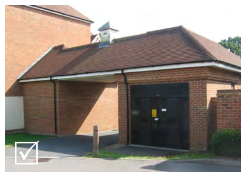
A carefully integrated sub-station accommodated at the entrance to a rear parking court which it helps to screen
