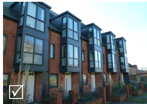
Dormers should be an integral part of the design and in proportion with the facade as in these town houses
