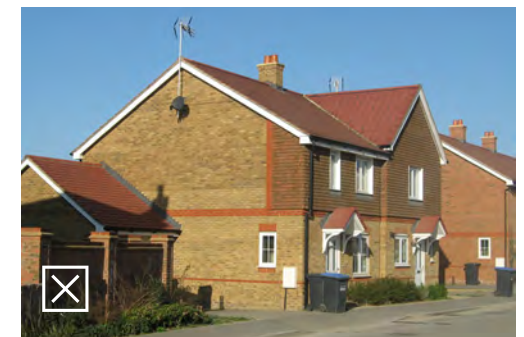
The clay hanging tile is inconsistently applied and appear to peel-away at the side. The roof tile also looks too bright in relation to the facing tile
