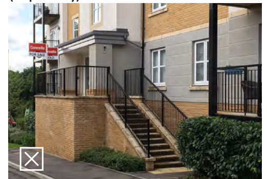
Elevating the entrance has divorced it from its street threshold and there appears to be no consideration for disability access
