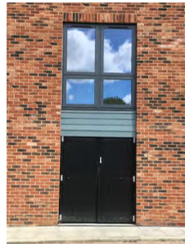
A bin store discretely accommodated within the façade
