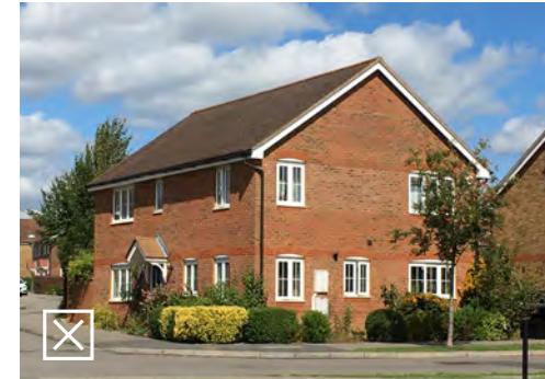
The lack of window articulation and absence of secondary facing material result in a bland façade. The elevations also suffers from inconsistently proportioned windows which incorporate fake glazing bars that undermine their authenticity
