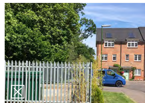
Pumping stations should be discreetly located where they don't impact negatively on the quality of the environment
