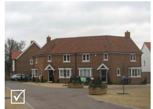
The chamfered corner ensures a continuous street frontage that overlooks and addresses the corner
