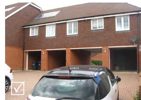
At the rear, the FOG provides direct natural surveillance over the parking court
