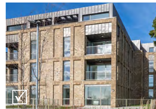
The elevations benefit from deep window reveals that add interest through the play of light and shade
