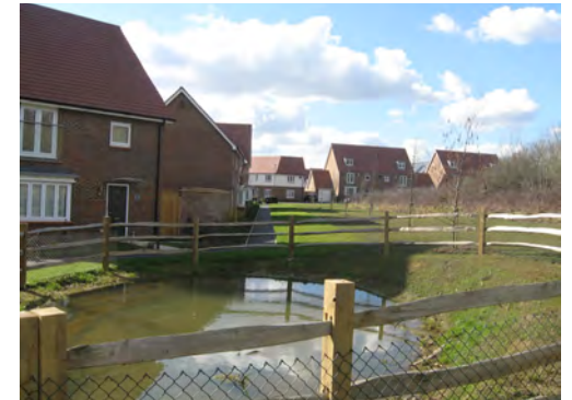
An appropriately domestic scaled attenuation pond
