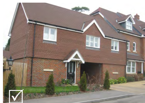
A FOG incorporating undercroft access to a rear parking court that is discreetly screened from the street by the building frontage
