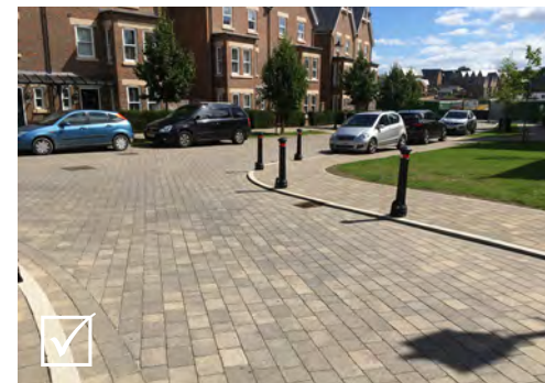
Imberhorne Lane, East Grinstead - high quality materials distinguish the shared surface areas
