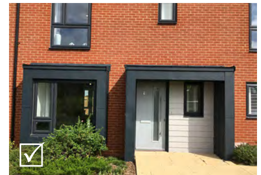
Entrances which are well defined by their canopies serving an apartment block and house (respectively)
