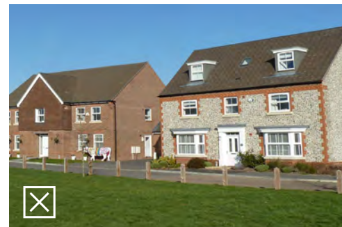
Poor pastiche design with a scale, proportions and detailing that fail to achieve a contextual response
