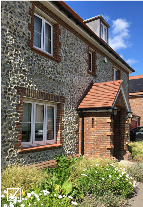
Flint facing combines well with brick detailing
