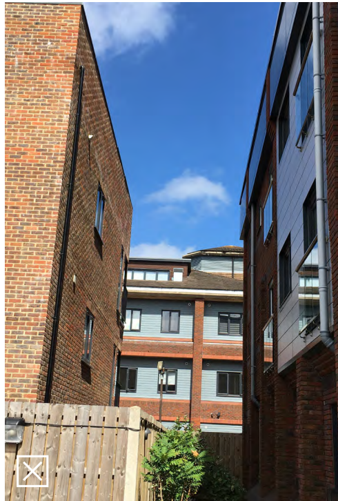
Buildings should be designed with sufficient separation distance to avoid privacy problems and a deficiency of daylight/sunlight
