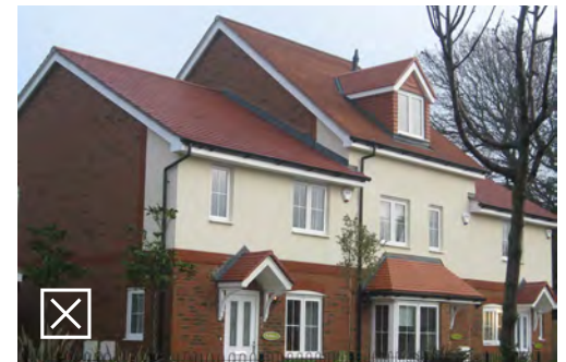
Clumsy juxtaposition of properties with inconsistent roof angles / over-dominant roof dormers
