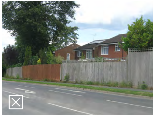
Houses that back on to the street unattractively expose their rear boundaries; this provides no animation or natural surveillance of the public realm while the gardens are subjected to traffic noise
