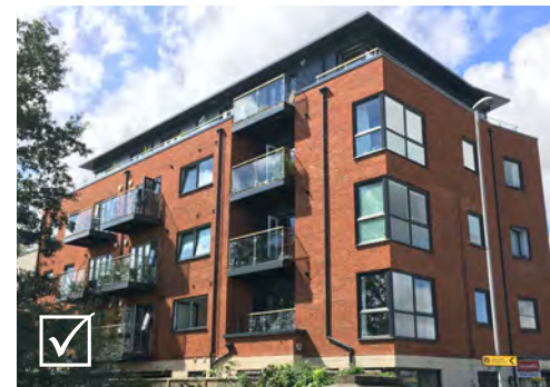
The set-back top floor helps to reduce the scale of this building
