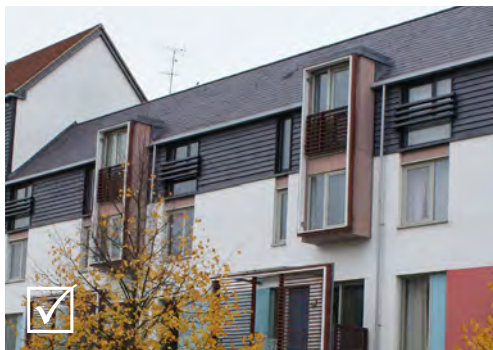
Dormers can be used in new development to reflect local vernacular in a modern way.
