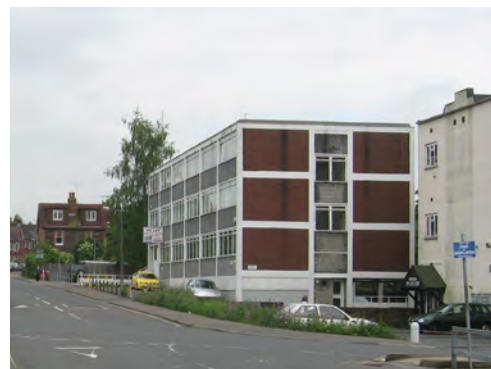
Office building in East Grinstead BEFORE conversion
