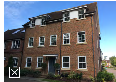
If not planned for rainwater downpipes can disrupt an elevation especially if it is otherwise symmetrically organised
