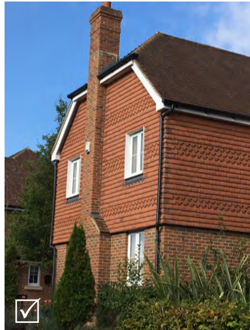
Natural clay hung (incorporating a beaver-tail pattern) tiles with local stock bricks and darker clay tiles employed on the roof
