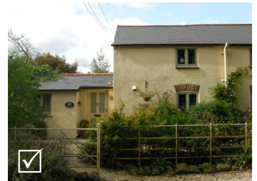
Successful single storey extension which is subservient to the original dwelling
