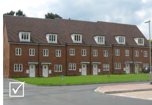
Rain water pipes have been positively accommodated to define the individual building frontages and thereby generate underlying rhythm
