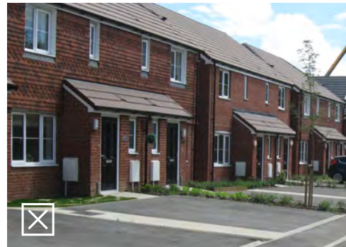
Meter boxes are prominent on building frontages
