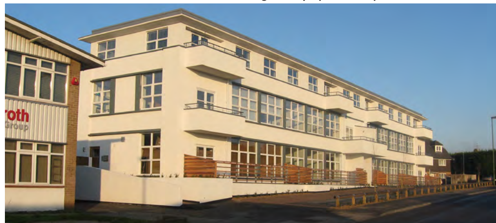
A sensitive residential conversion of an Art Deco style commercial building incorporating an additional storey
