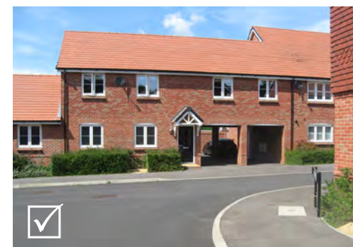
Undercroft tandem parking is space efficient and discreet enabling strong street enclosure
