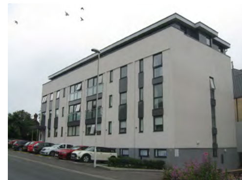
Office building in East Grinstead AFTER conversion. Whilst there are still some issues with the public realm treatment the scheme is generally a positive improvement
