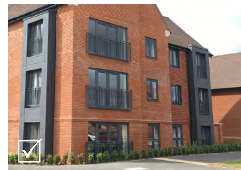
Juliet balconies can add interest to facades while providing rooms with a greater connection to the outside
