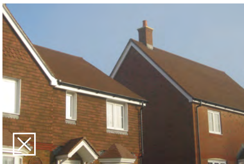
Fake chimneys should normally be avoided as they often look unconvincing and undermine architectural integrity
