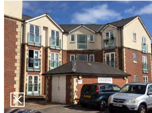
Bin store obscures building frontage and presents a poor outlook from properties
