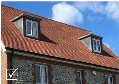
Dormer windows should be suitably sized and proportioned so that they are subservient to the roof
