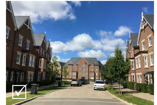
Strong street enclosure provided by consistent building lines and 3/4 storey frontages
