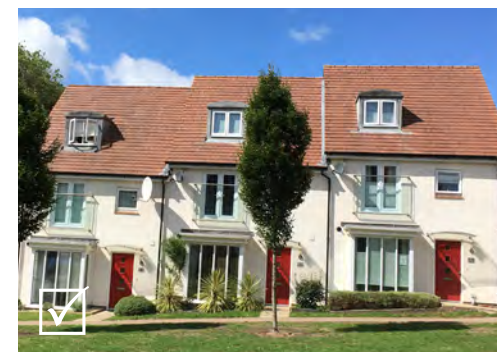
Windows have been carefully organised in a logical hierarchy that graduate in size from the ground floor to the top floor
