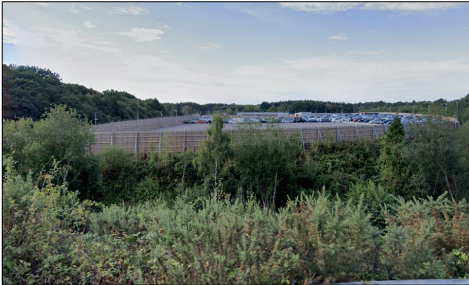
Figure 15 - Airport related parking recently constructed in the plan area.
