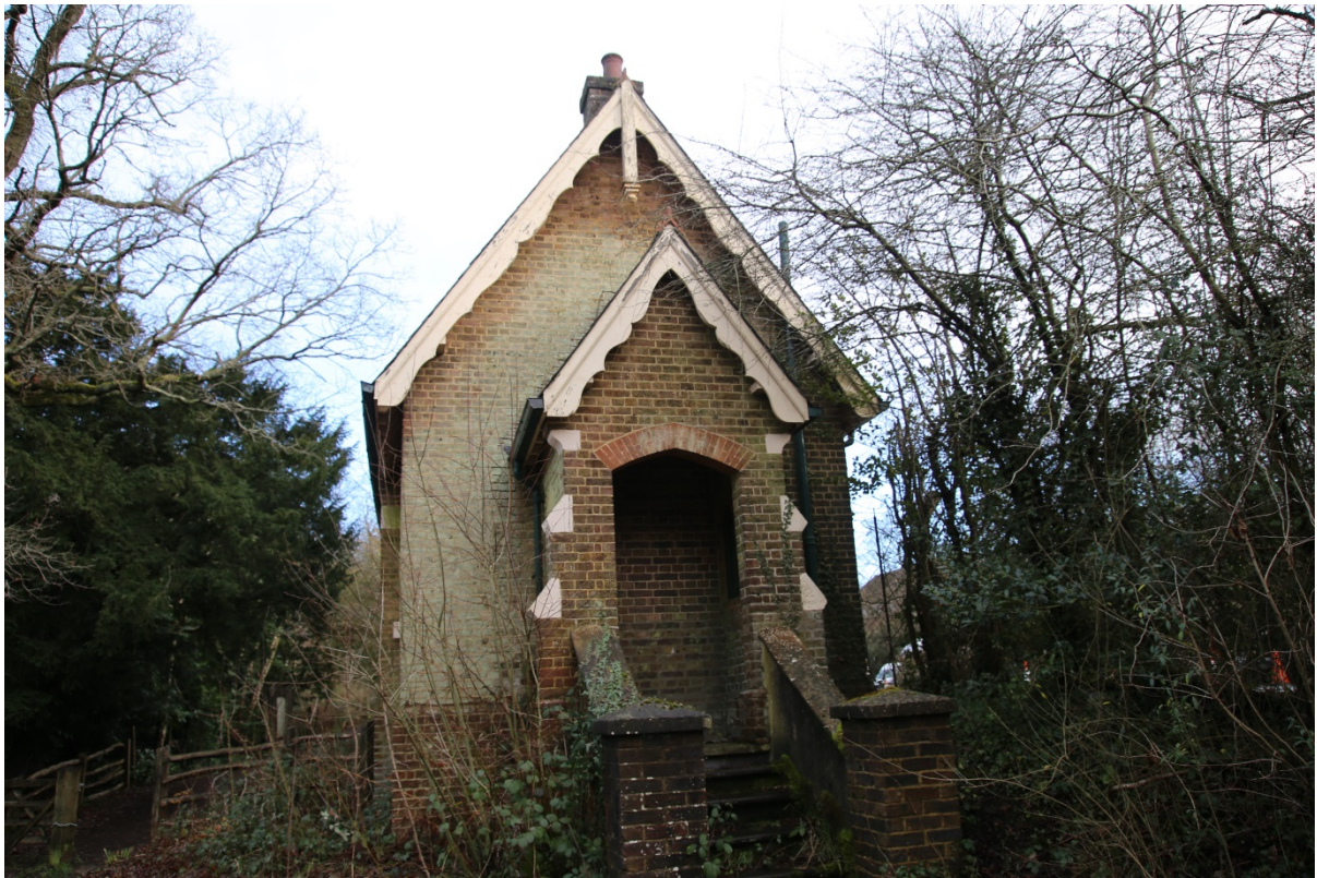
Rowfant Estate shelter at Railway Station
