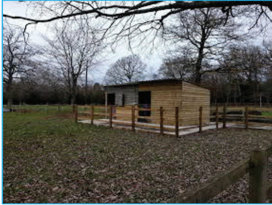
Photo 1 Stable building (B1)-negligible suitability for roosting bats
