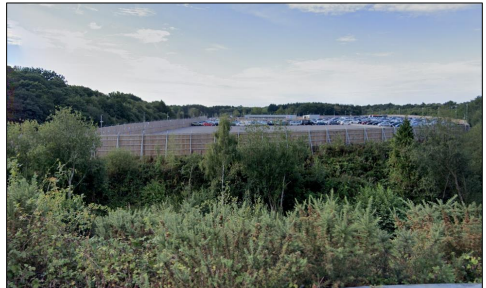
Figure 13 - Airport related parking recently constructed in the plan area.
