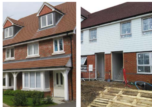
Poor quality modern versions of these details and materials
