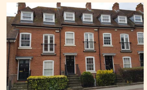
These apartments have been designed to appear as terrace houses in the street scene, with each front door serving two apartments
