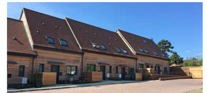
This contemporary styled housing development has successfully used steep roof pitches, stepped terraces responding to the site's topography, a strong building line and a variety of unit frontage widths
