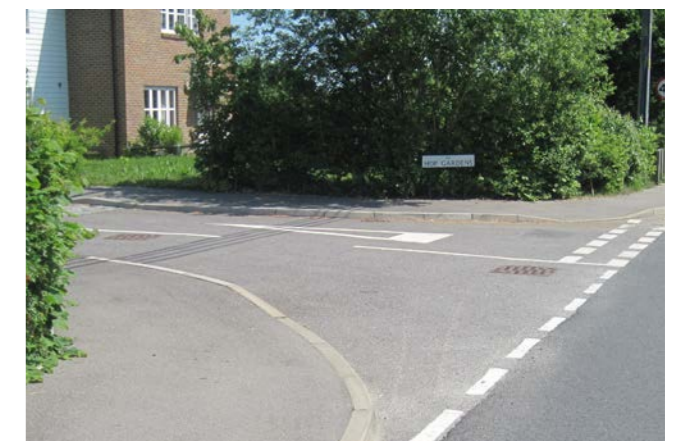
These two road junctions access similar numbers of houses. However, the top image shows a clearly subservient road, reflecting its hierarchy, with tight radii, no white lines, a simple pavement picked out by a small kerb, and traditional materials. In contrast, the image below shows a visually engineering-heavy approach, contrary to MfS and inappropriate for this scale of development in a rural context in the High Weald
