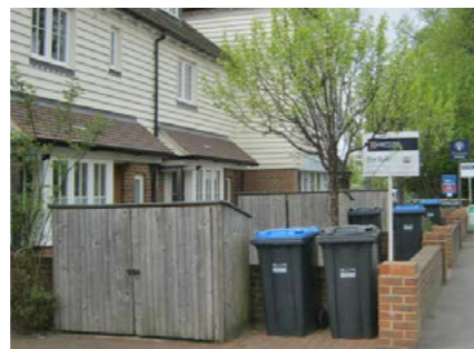
Conversely, the strong building detailing of this scheme is undermined by the forecourt clutter of bins and stores creating a poor streetscene
