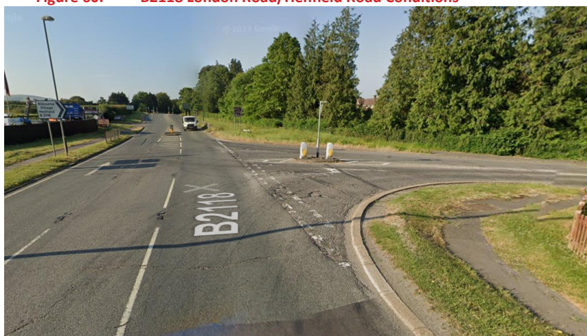
Figure 60. B2118 London Road/Henfield Road Conditions
