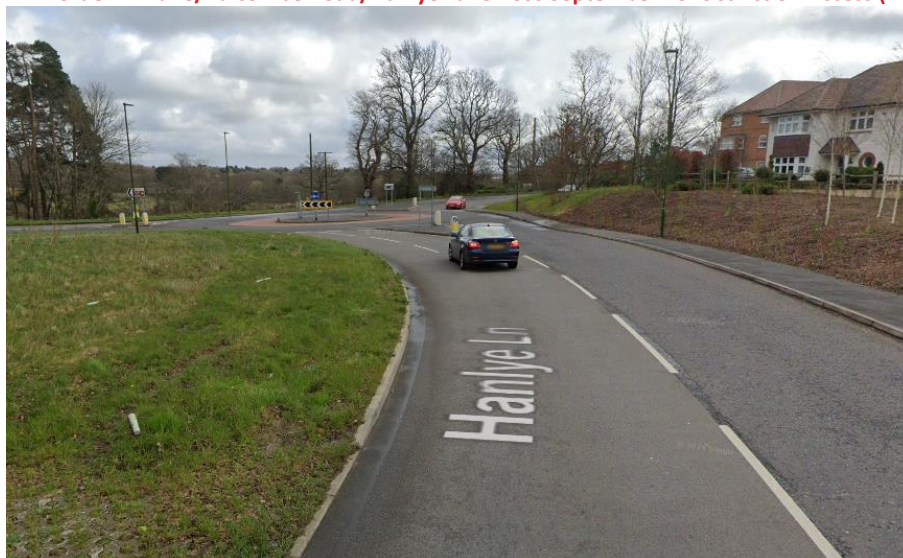
Figure 5. Borde Hill Lane/Balcombe Road/Hanlye Lane Post-September 2020 Junction Access (Western Arm)
