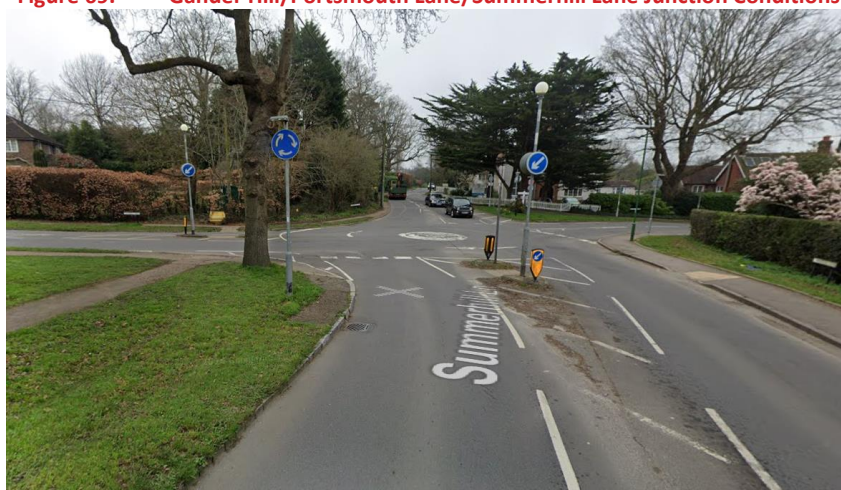
Figure 69. Gander Hill/Portsmouth Lane/Summerhill Lane Junction Conditions
