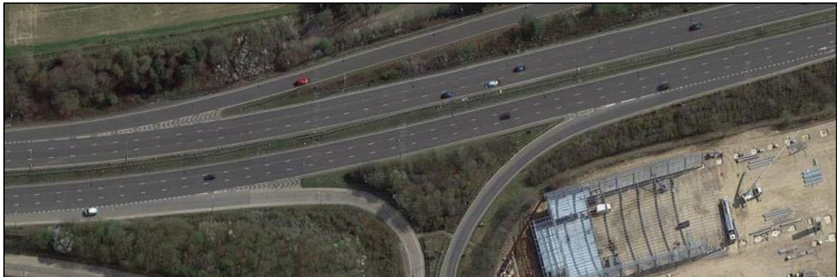
Figure 79. Aerial View of A23 A272 Northbound Slips and Southbound Off-slip
