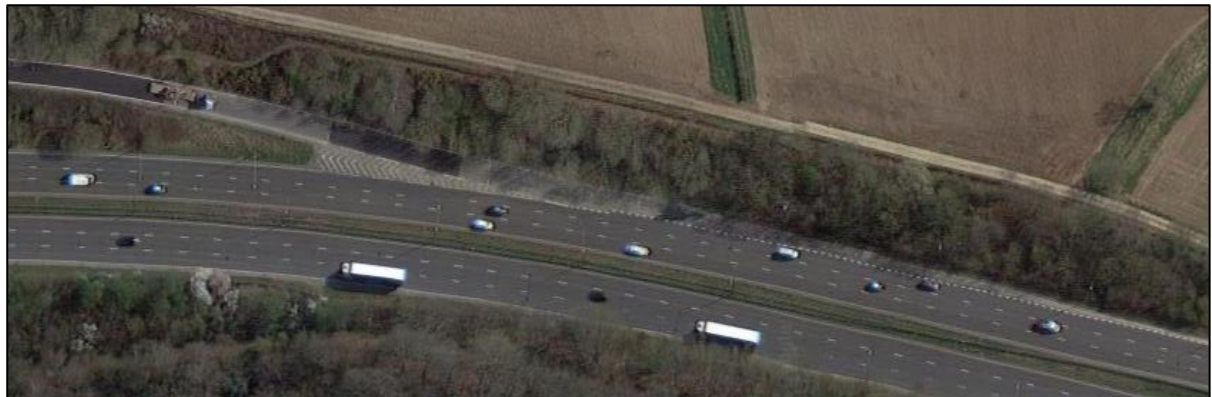
Figure 80. Aerial View of A23 A272 Southbound On-slip
