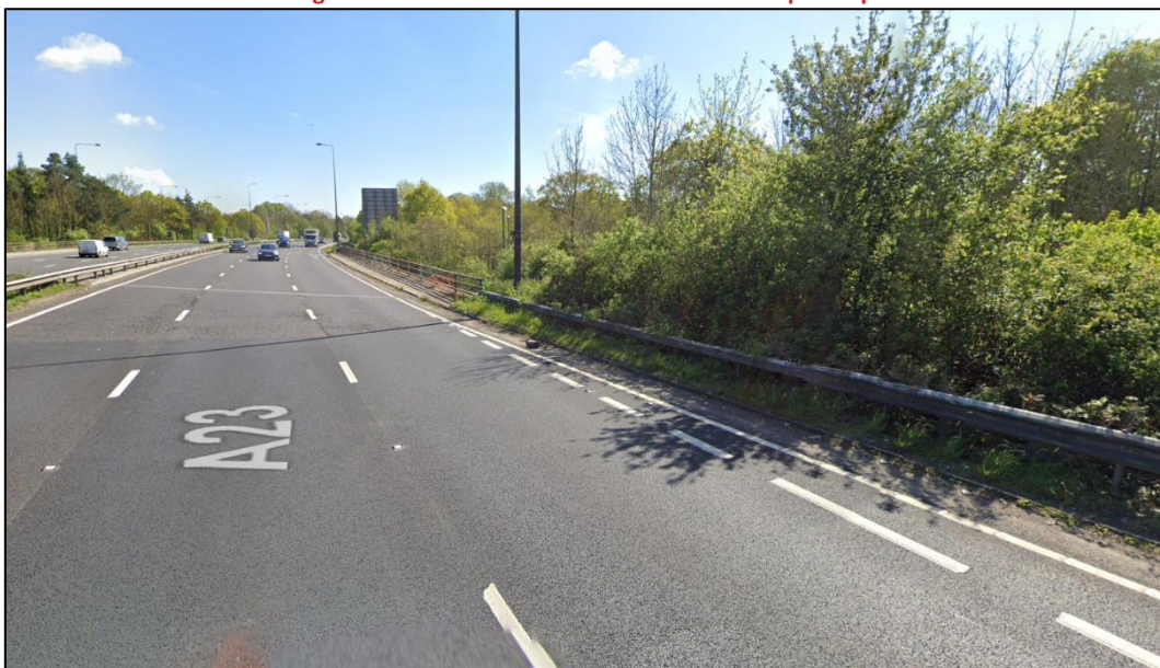
Figure 84. A23 A272 Northbound Off Slip Overpass
