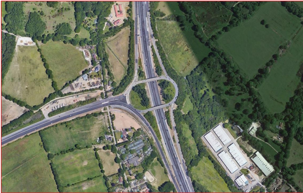
Figure 3. Aerial view of M23 Junction Layout
