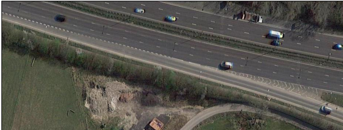
Figure 71. Aerial view of A23 Broxmead Lane Northbound On-slip
