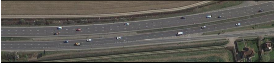
Figure 94. Aerial view of A23 A2300 Northbound Merge Layout
