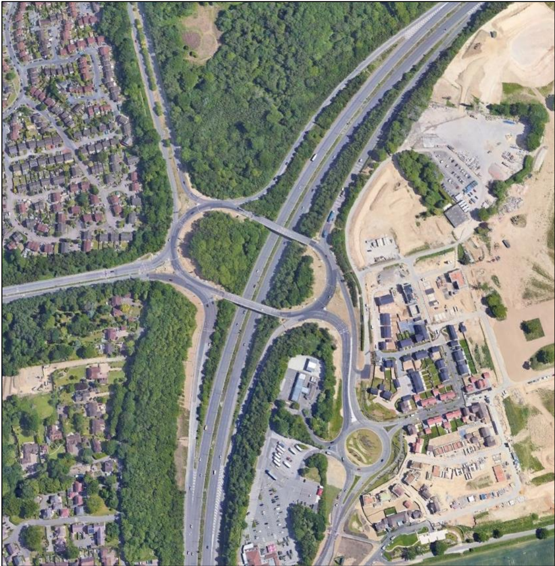
Figure 32. Aerial view of M23 Junction 11 Layout
